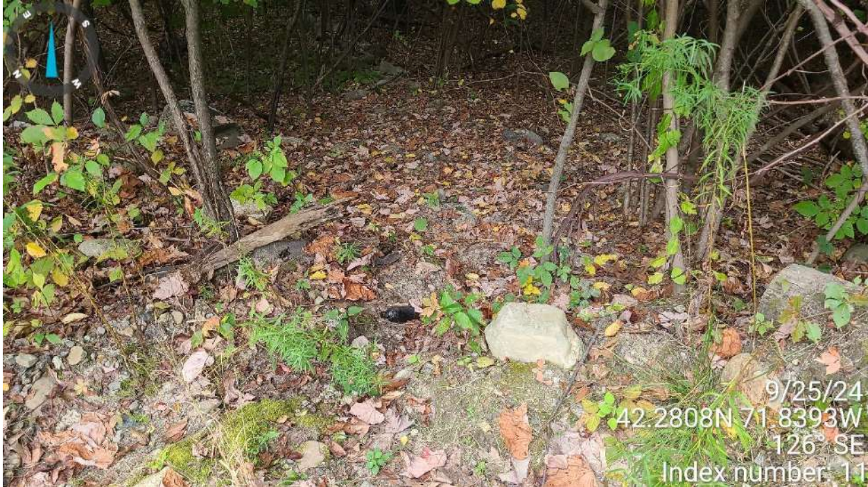
Photo 4: Toe of slope facing southeast at property line (lowest point).
